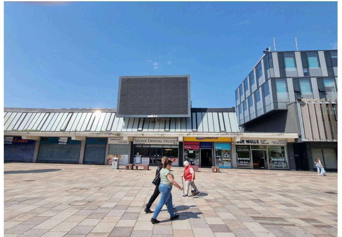
Increasingly, the town centre has multiple vacant and empty units impacting on town centre appeal.
