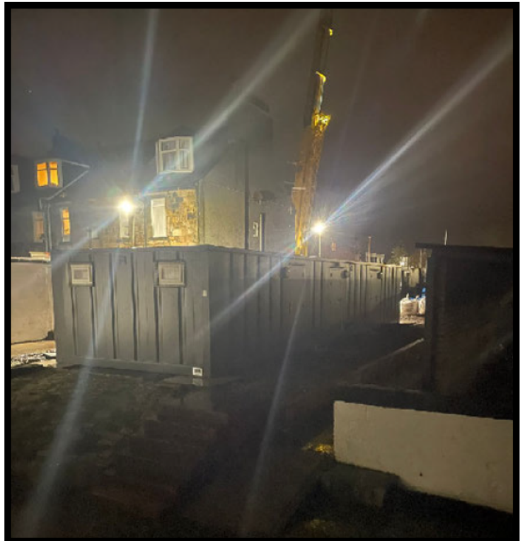
THE NEW BLOCK BEING CRANED INTO POSITION
