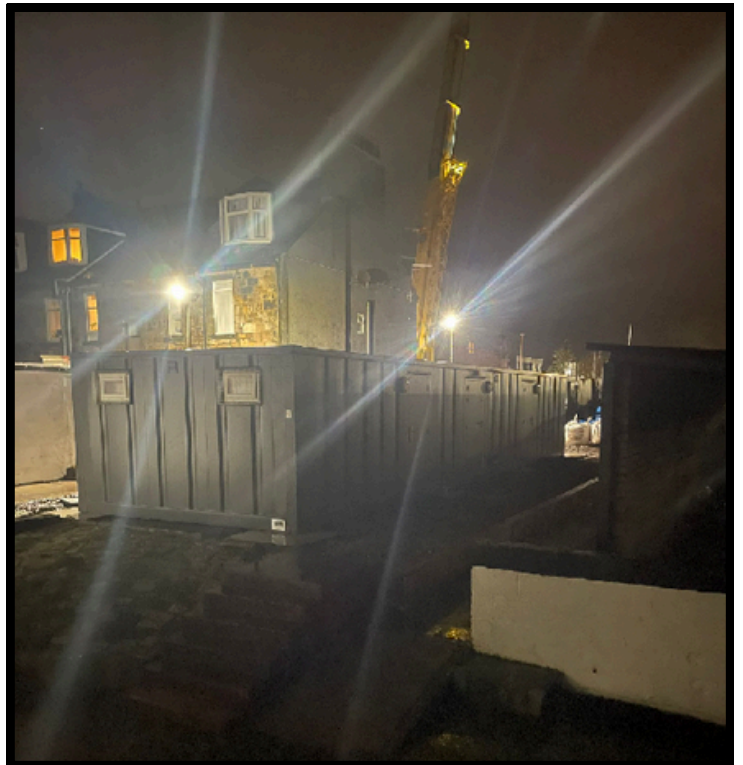
THE NEW BLOCK BEING CRANED INTO POSITION
