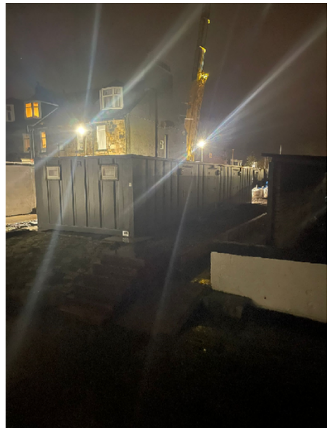
The new changing facility being craned onto site
