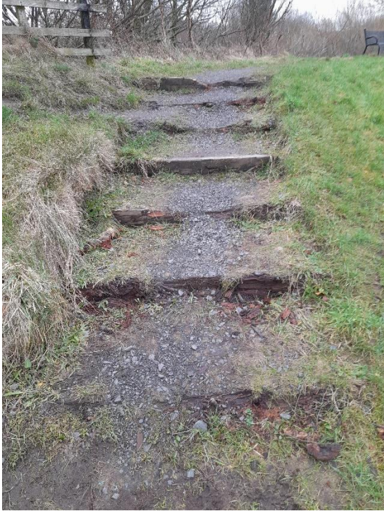
Steps before work started
