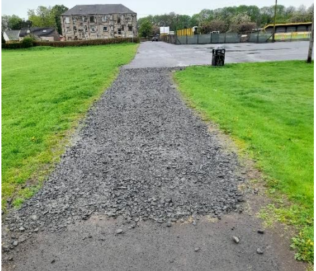
Path between bridge and car park
