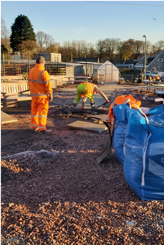
Staff from DAMM lay the slabs donated by McLaughlin and Harvey
