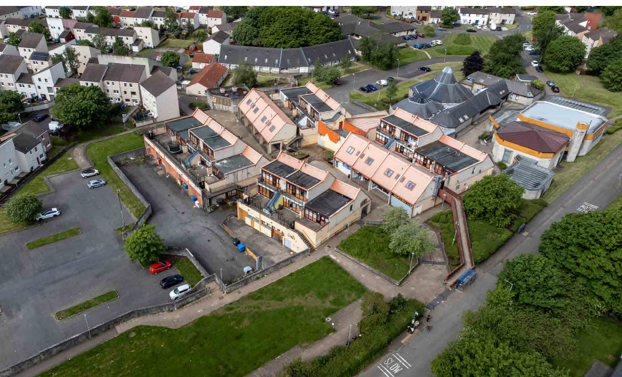
Aerial View Looking West
