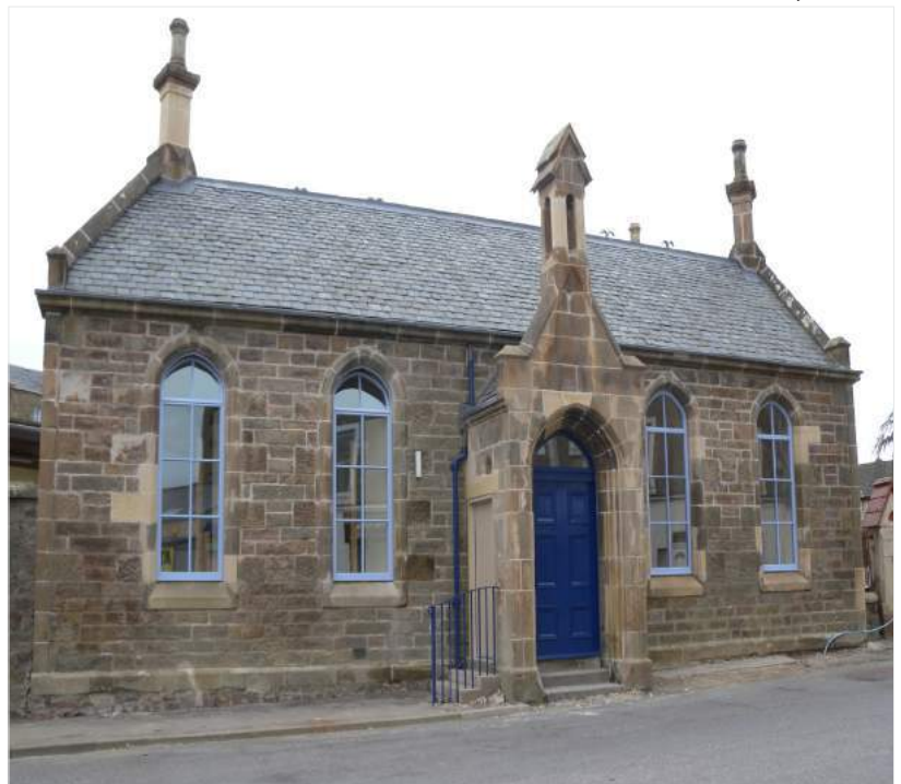
Slimline double-glazed windows improve energy efficiency and meet conservation requirements
