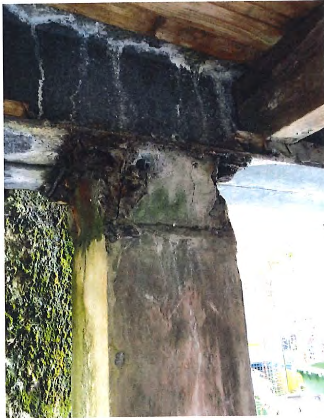
Southeast elevation/undercroft - Damaged steelwork
