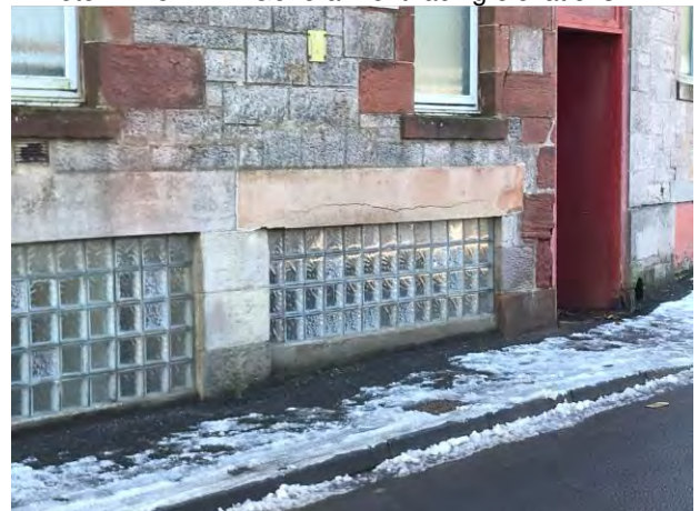
Photo 10. Cracking across lintel to basement windows
