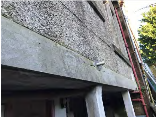
Photo 13. General cracking to structure of south-east extensions
