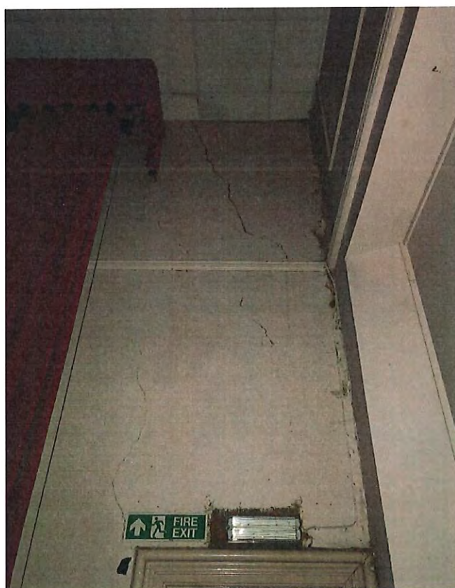
Main hall rear wall (Southwest gable) - cracking
