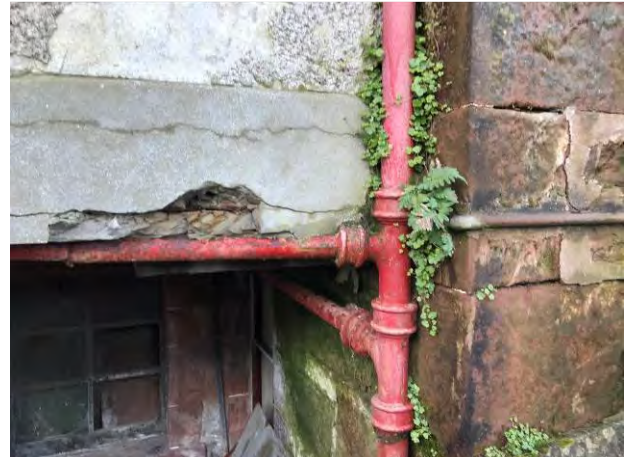
Photo 14. Corrosion to embedded steelwork
