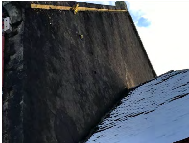
Photo 3. Cracking to high level render
