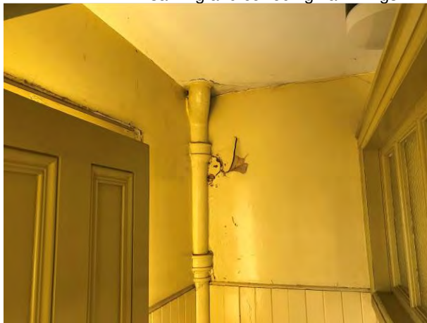
Photo 21. Water damage around downpipe
