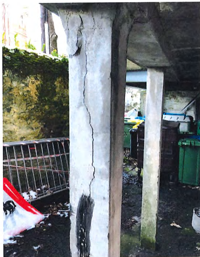
Southeast elevation - Damaged support columns
