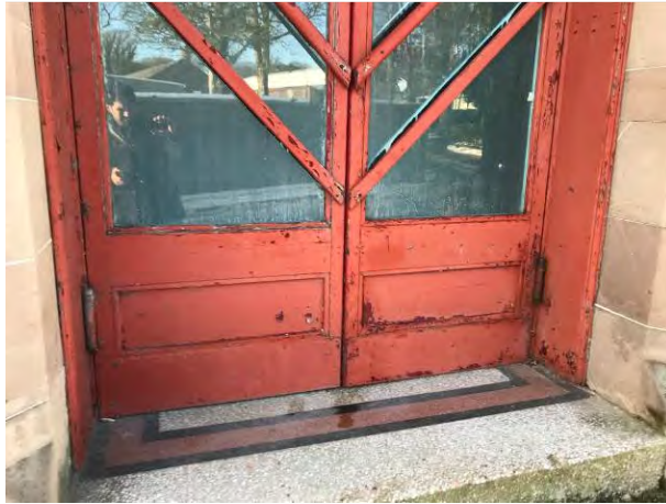
Photo 7. Timber decay to front doors
