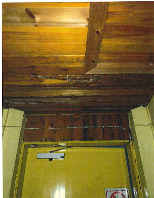
Ground floor hallway - Water ingress/dampness
