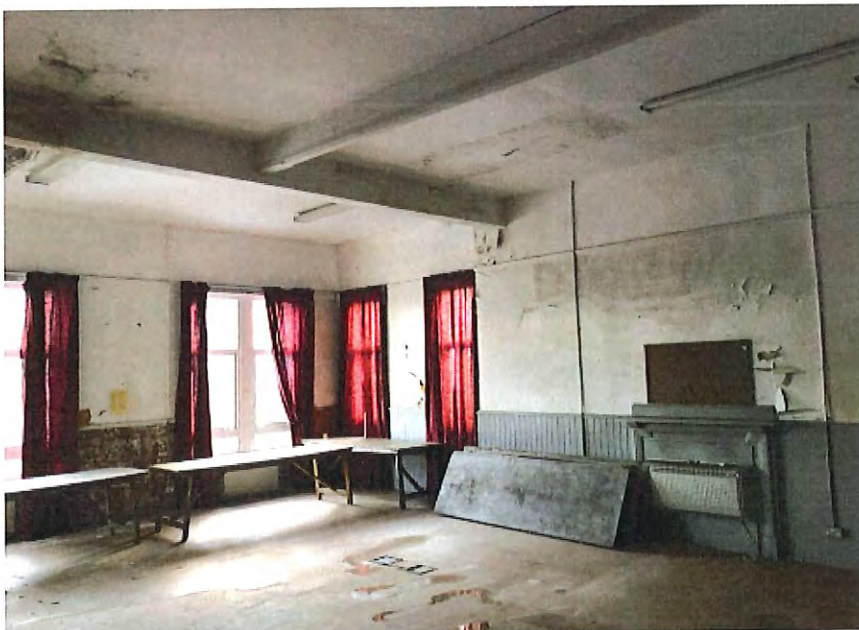
Small rear hall - Water ingress/dampness & damage
