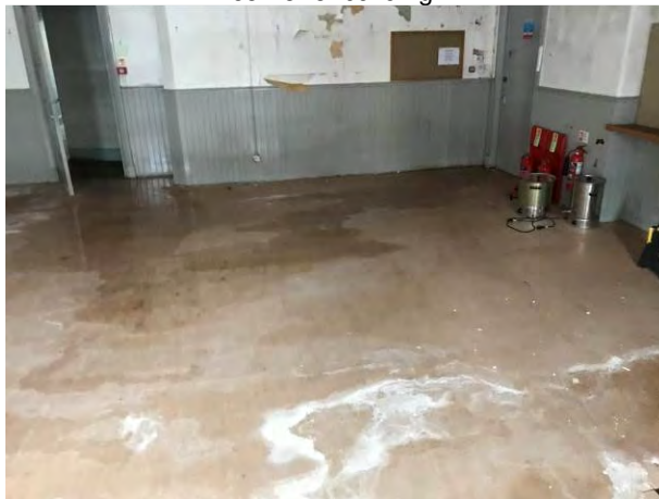
Photo 27. Severe water ingress/damage within room 0/012
