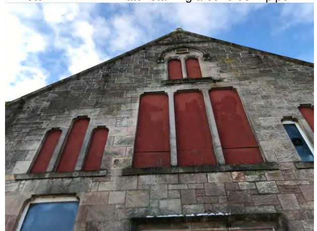
Photo 6. Previous mortar repairs to front elevation
