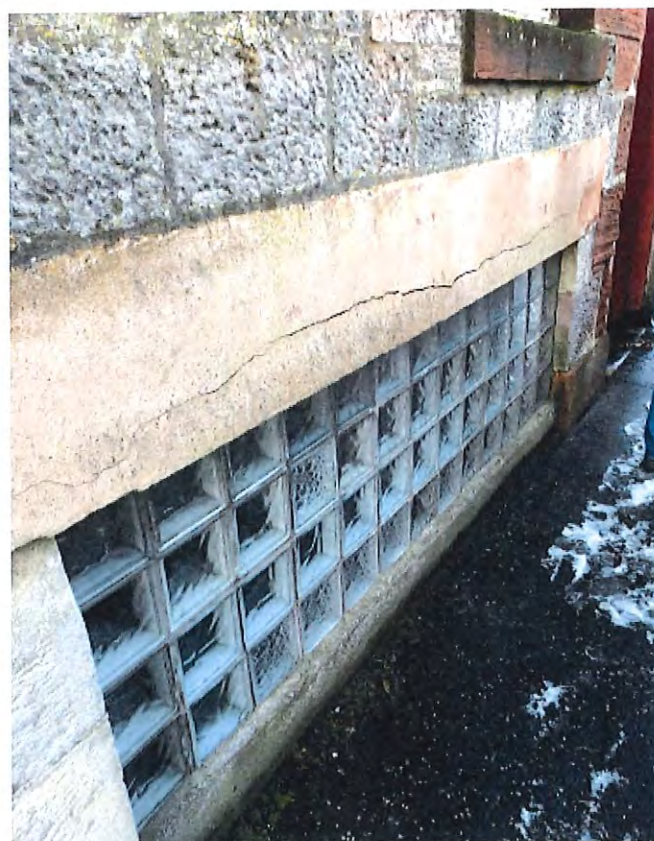
Clifton Street elevation - cracking across lintels
