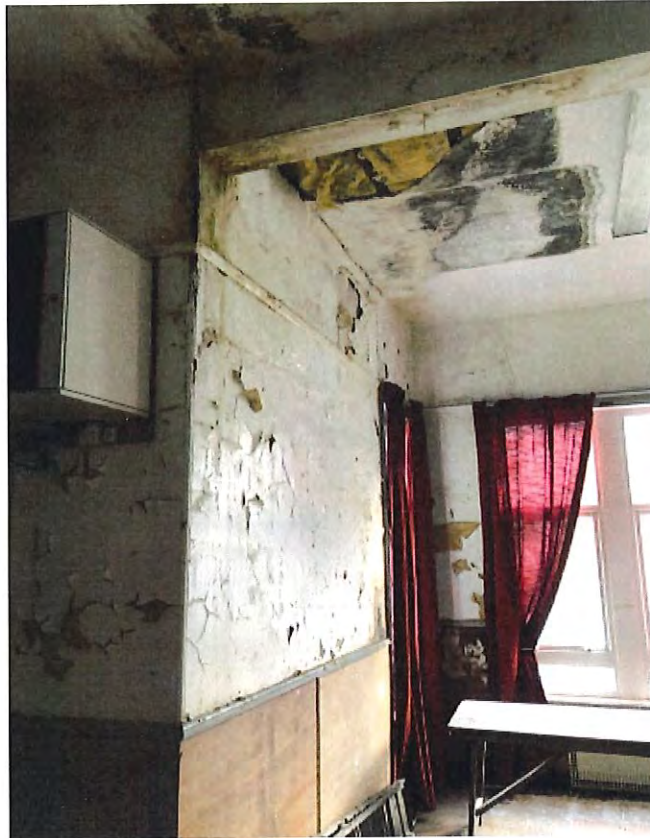
Small rear hall - Water ingress/dampness & damage
