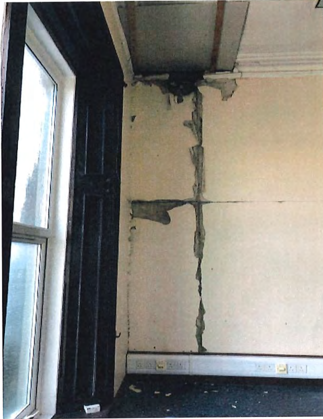
Small hall (along Clifton Street) - Water ingress/dampness
