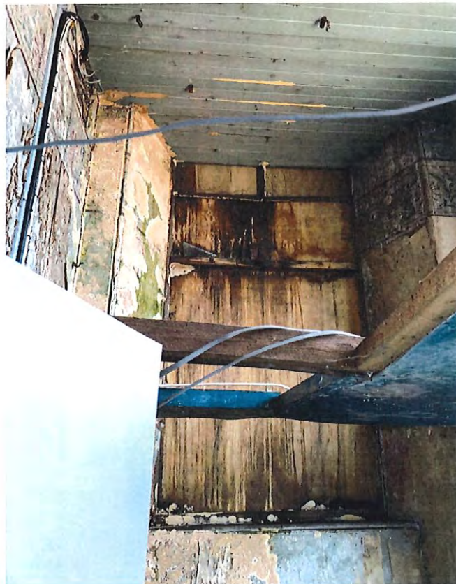
Main hall (Howard Street elevation) - Water ingress/dampness
