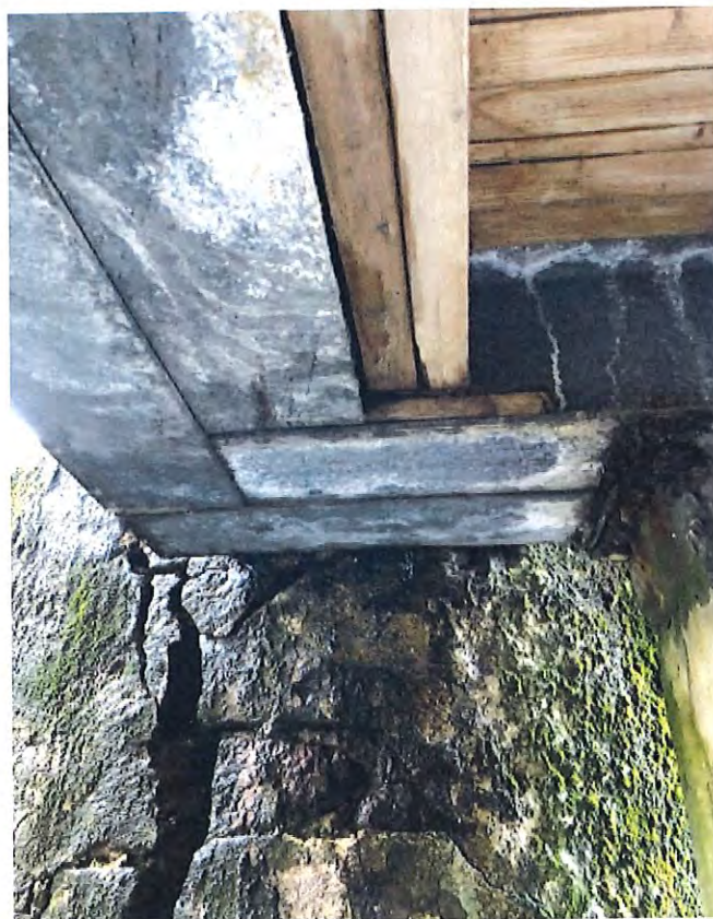
Southeast elevation/undercroft - Damaged masonry
