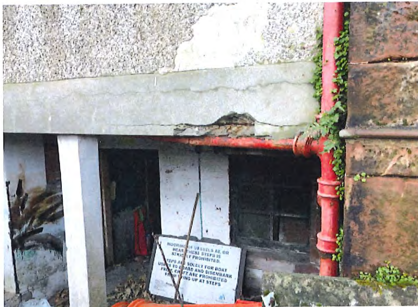
Southeast elevation - Damaged steelwork, concrete & masonry
