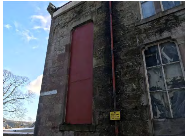
Photo 4. Water staining around downpipe
