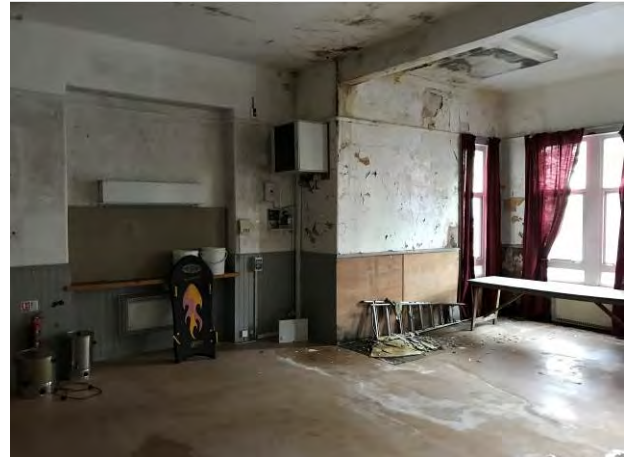
Photo 26. Severe water ingress/damage within room 0/012
